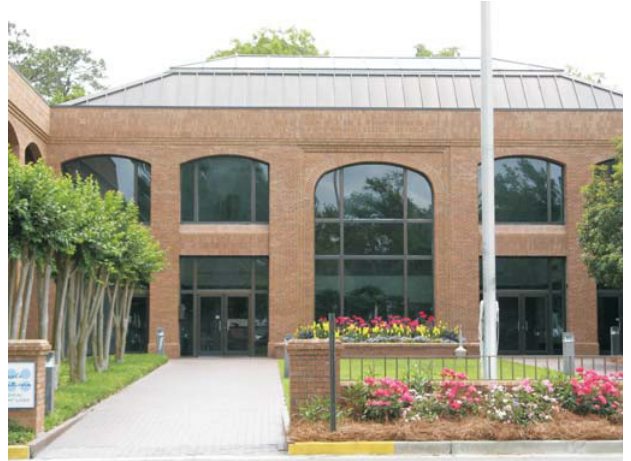
The Southside's 6602 Abercorn Building
